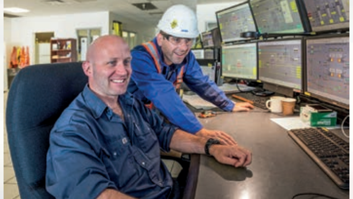
Christoph Gruber, Commissioning Manager from ANDRITZ (standing), with Trevor Turner, Head Boiler Operator, in the control room. ▶
