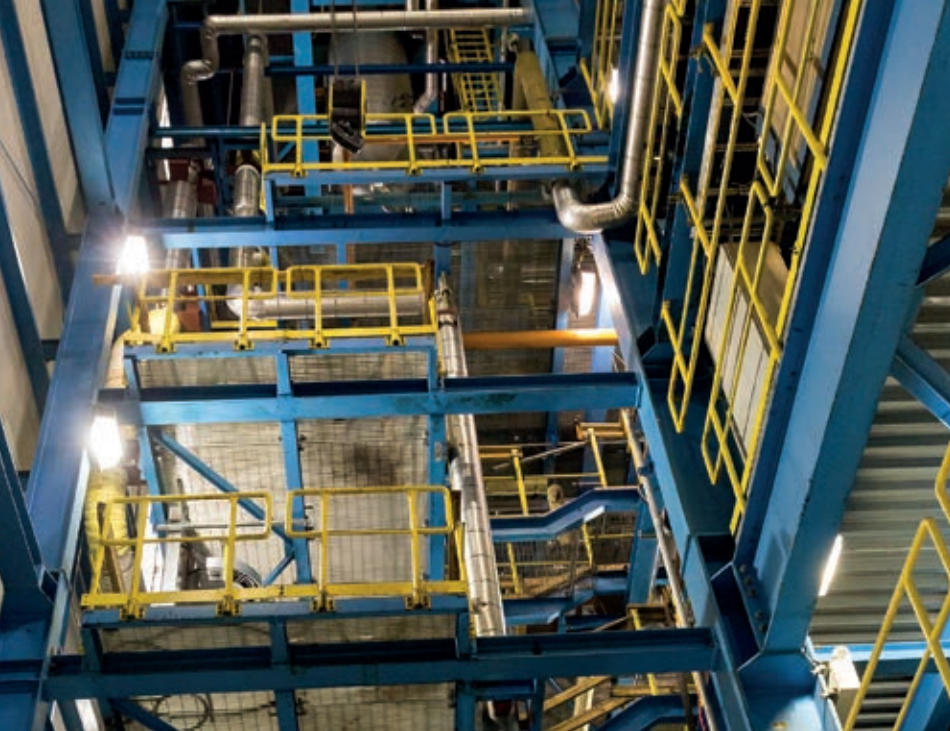
▲ The ANDRITZ boiler has capacity to burn 78.5 t of wet liquor at 50% dry solids each hour, equating to 942 tds/d producing 222 t/h of high-pressure steam.
