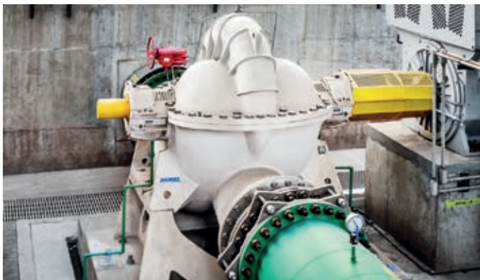
◀ These low-maintenance pumps have been optimized for use in the pulp and paper industry, where they operate with an efficiency of over 90% with low pulsation.
