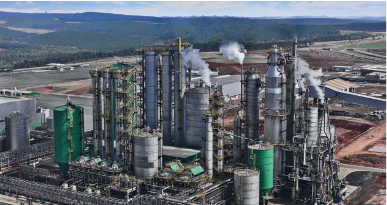
▲ ANDRITZ delivered two fiberlines for the mill: a 1.1 million t/a hardwood line and a 400,000 t/a softwood line. Much of the softwood will be used for the production of fluff pulp.
