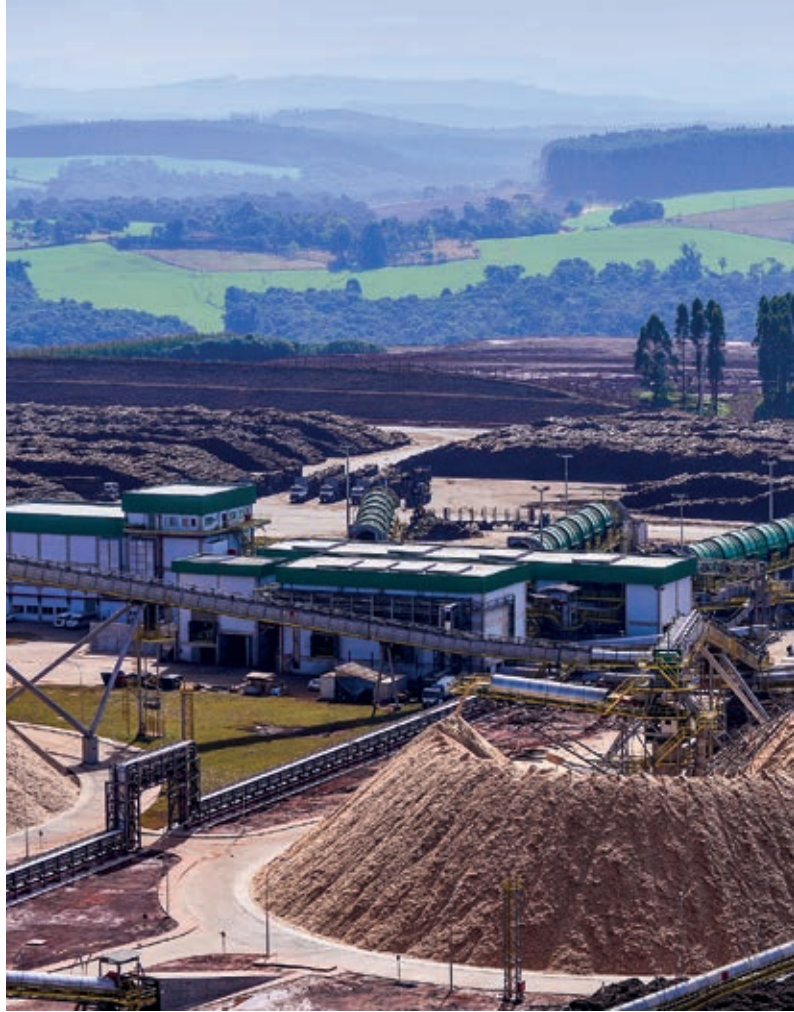
Overview of the ANDRITZ woodyard with one of the two 360° stacker reclaimers in the foreground and four chipping lines in the background. ▶
