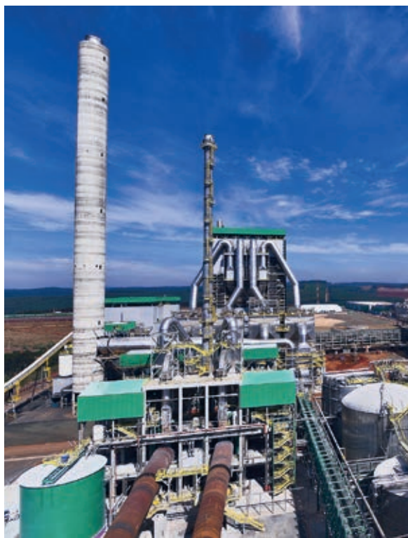
◀ In the white liquor plant, there are two kilns (capacity 650 t/d each). The recausticizing plant is designed to produce 16,000 m 3 /d.
