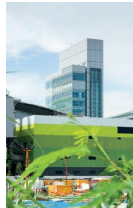
▲ The power plant uses four EcoFluid boilers (bubbling fluidized bed technology), arranged in two sets, to incinerate the incoming sludge. Each has a 14 MW steam turbine.
