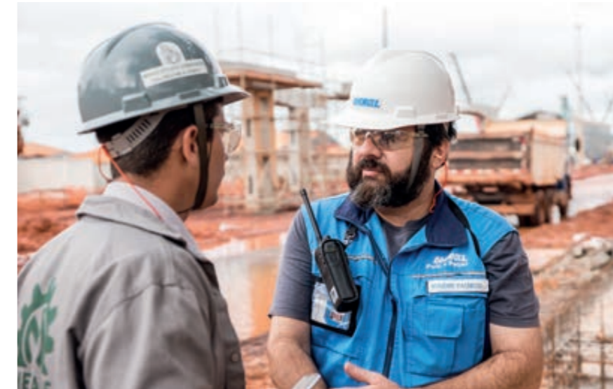
Rogério Pacheco, Fiberline Site Manager, talks with a supervisor from the mechanical erection company. ▼
