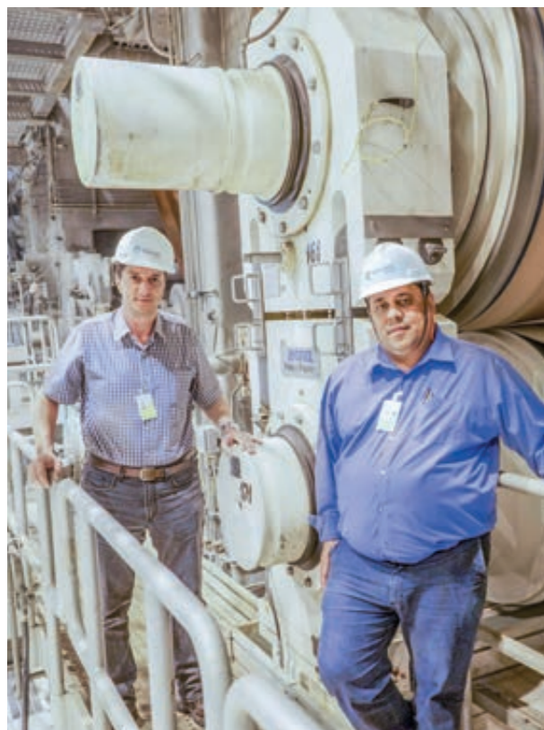
◀ Ademilson Zeber, Drying Coordinator, (left) with Josué Fernandes, Coordinator for Packaging and Logistics, at the press section of one of the two high-capacity dewatering machines.
