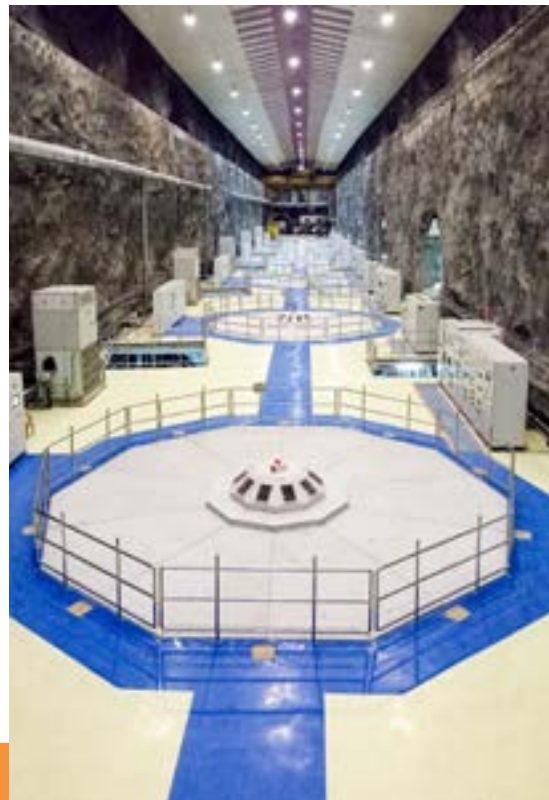
Teesta Stage III, Teesta River, 1,200 MW
