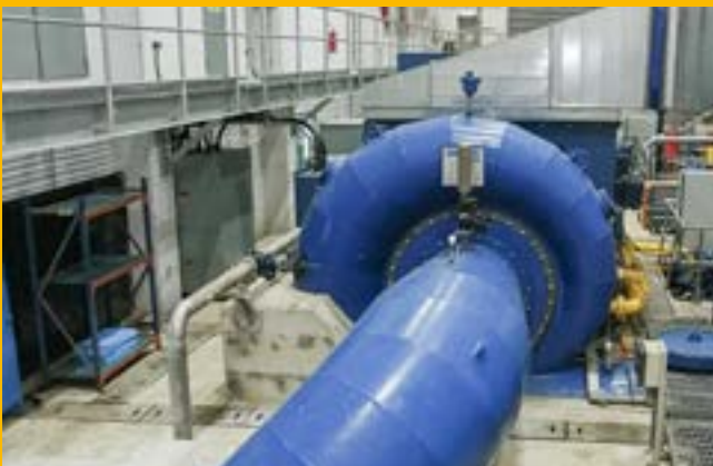
Tembat Station, Hulu Terengganu hydroelectric project, Sg. Tembat Tributary, 2 × 7.5 MW
