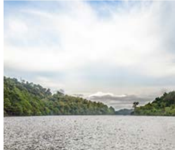
Kaptai Lake near Karnafuli, Kaptai Dam, 6 × 48 MW
