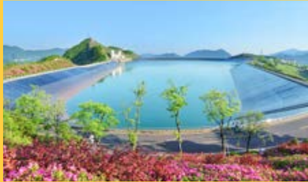
Tian Huangping pumped storage plant, Zhejiang Province, 6 × 306 MW
