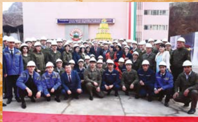
Nurek, Vakhsh River, Tajikistan, 3,420 MW Grand official ceremony for the start of the rehabilitation program
