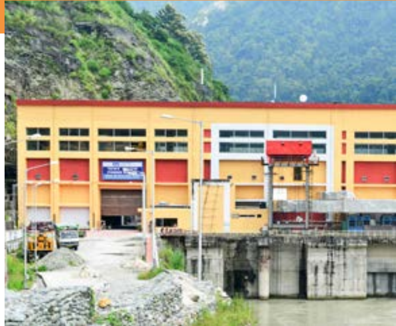
Teesta Low Dam Stage III, Teesta River, 132 MW
