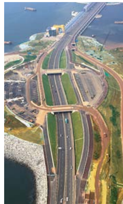
Sihwa tidal power plant, Sihwa Lake Dam
