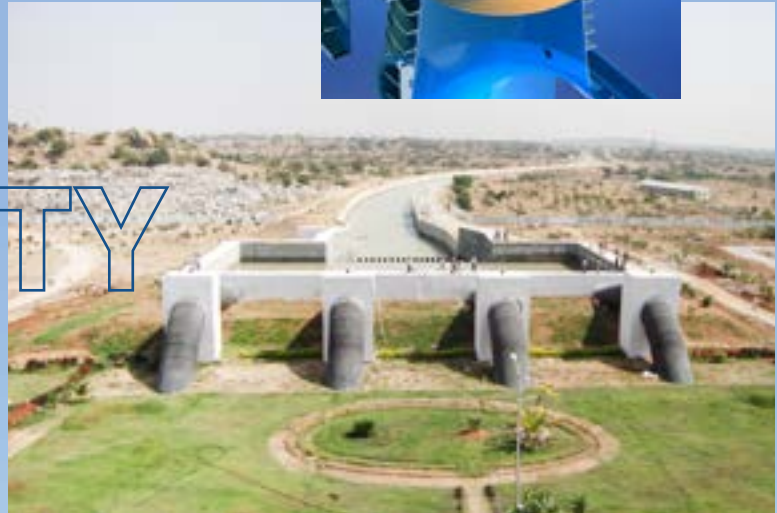
Bheema pumping station, three vertical volume pumps
