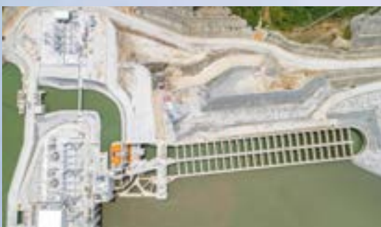
Fish ladder, Xayaburi hydropower plant, Lao PDR
