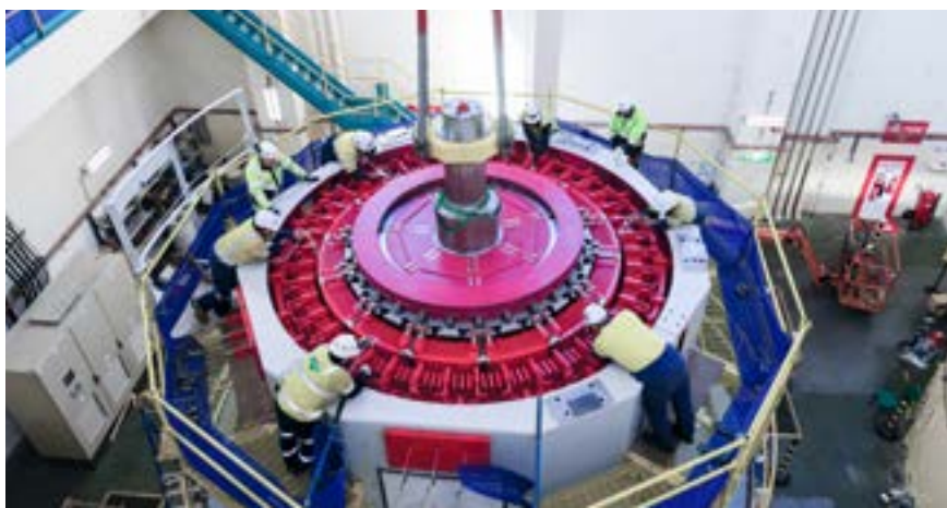
Installation works, Guthega, New South Wales, 45 MVA
