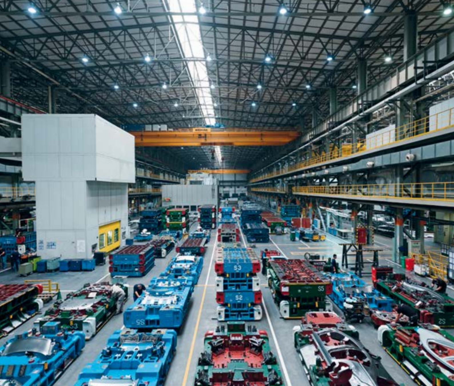
The new FAW-Volkswagen press hall in Changchun, China, measures almost 26,000 square meters and is 20 meters high. After all, it needs to be big enough for up to three huge Schuler press lines to manufacture various car body components.
