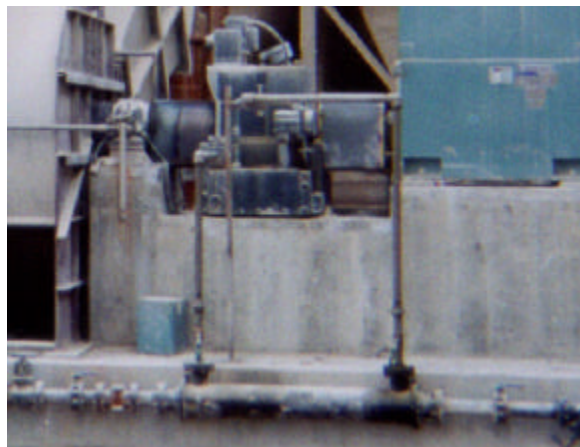
Fig. 3. Fluid Coupling Installation
