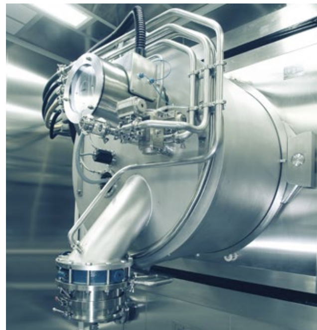
Clean room installation
